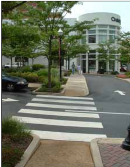
Clearly marked crosswalks, corner “bulges”, and handicapped curb cuts welcome pedestrians and increase safety
